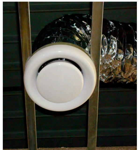
4. Insert Grille...After Ceiling is installed.
