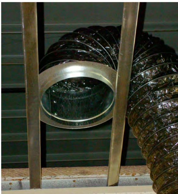
3. Secure Into Trusses & Add Flex
